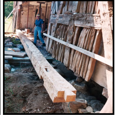
Base beam ready to be laid. 2007
