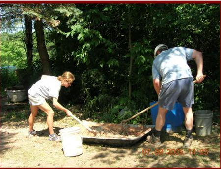
**Station 4** was the “sand pile and water barrel”. Sand and water are added to the mixture. Sand was shoveled into buckets and taken to the mixer.
