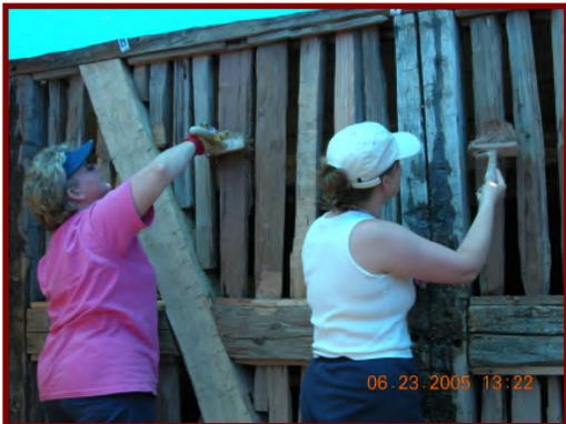
**Station 6** was the “Slurry Painters”. Fine clay was mixed with water to a paint-like liquid and painted on the staves and inside of timbers so the nogging would stick better. Those who “painted”
