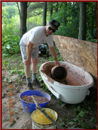
**Station 2** was “the bath tub”. A discarded fiberglass bathtub shaped hot tub donated to CS was used to reconstitute the clay. Water was added to the dry clay. Now, “Why?”, you ask, “did we dry it only to make it wet again?” The clay particles all must be equally dry and then moistened to have a mud mixture that will dry in the walls evenly. If not, it will crack and fall out.
